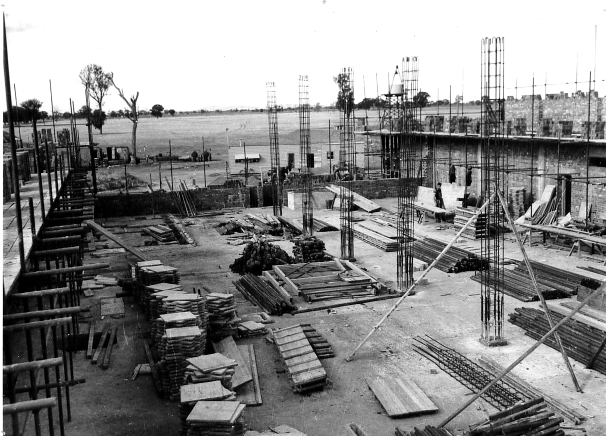
The brick and concrete work of the transmitter building 1943
