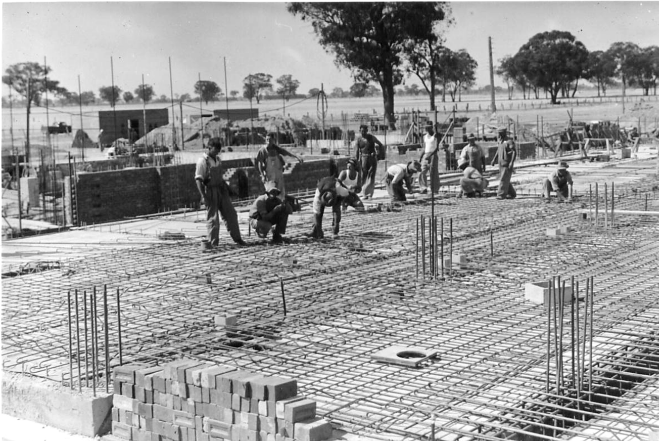
Transmitter Hall Floor March 1943 basement already in
