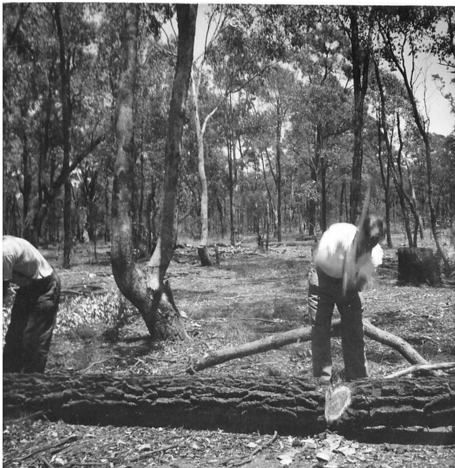
Cutting a timberpole for transmission lines
