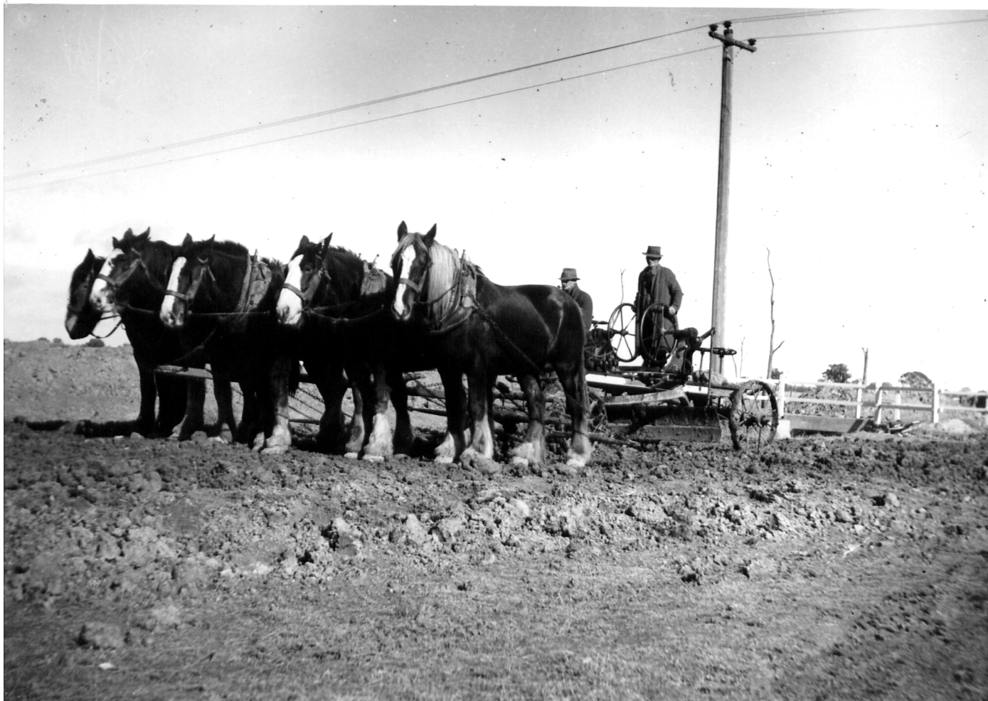
Horses and grader filling in control cable trenches 1943 / 1944
