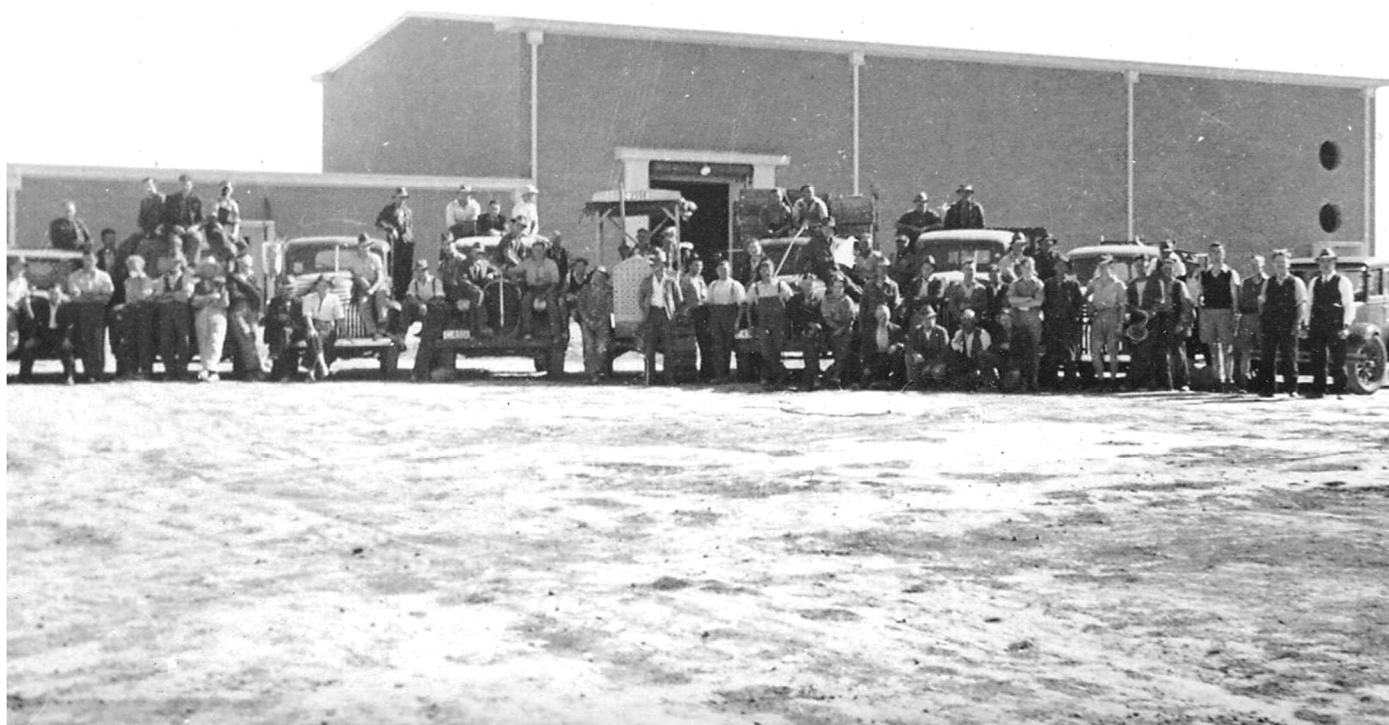
Assembled at the completion of the building on the site
