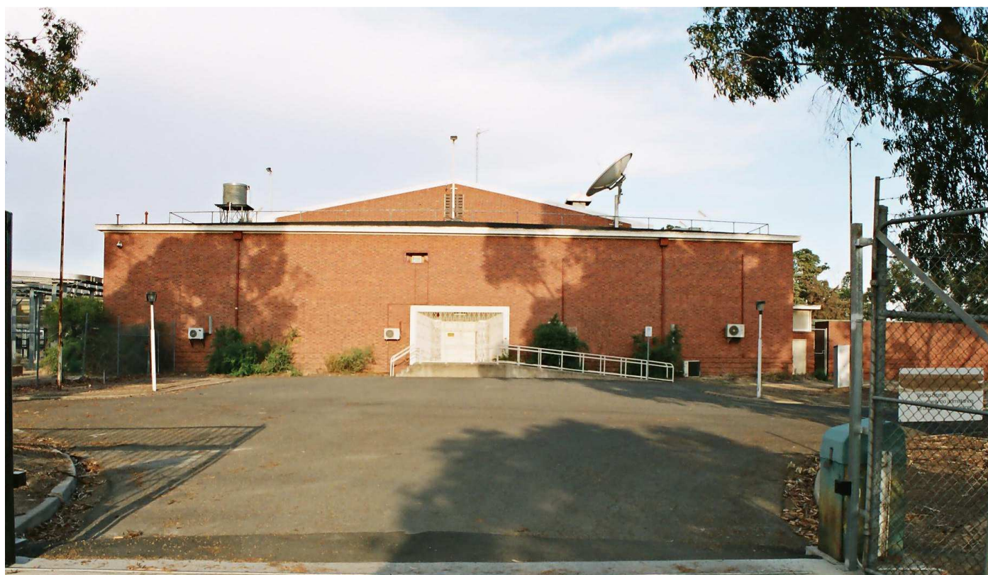
Front gate entrance 2007
