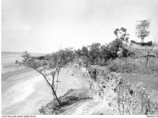
1942 - The first radar station aerial (background) installed in Darwin is camouflaged to look like a tree. It was the first in Australia to give warning of approaching Japanese raids. (AWM)
